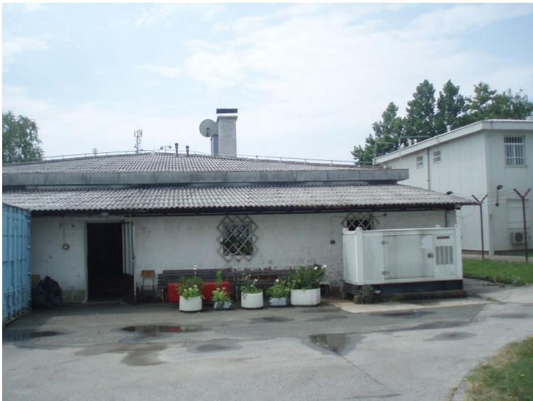
Pitcure No. 2 - existing kitchen premises that will be reconstructed
